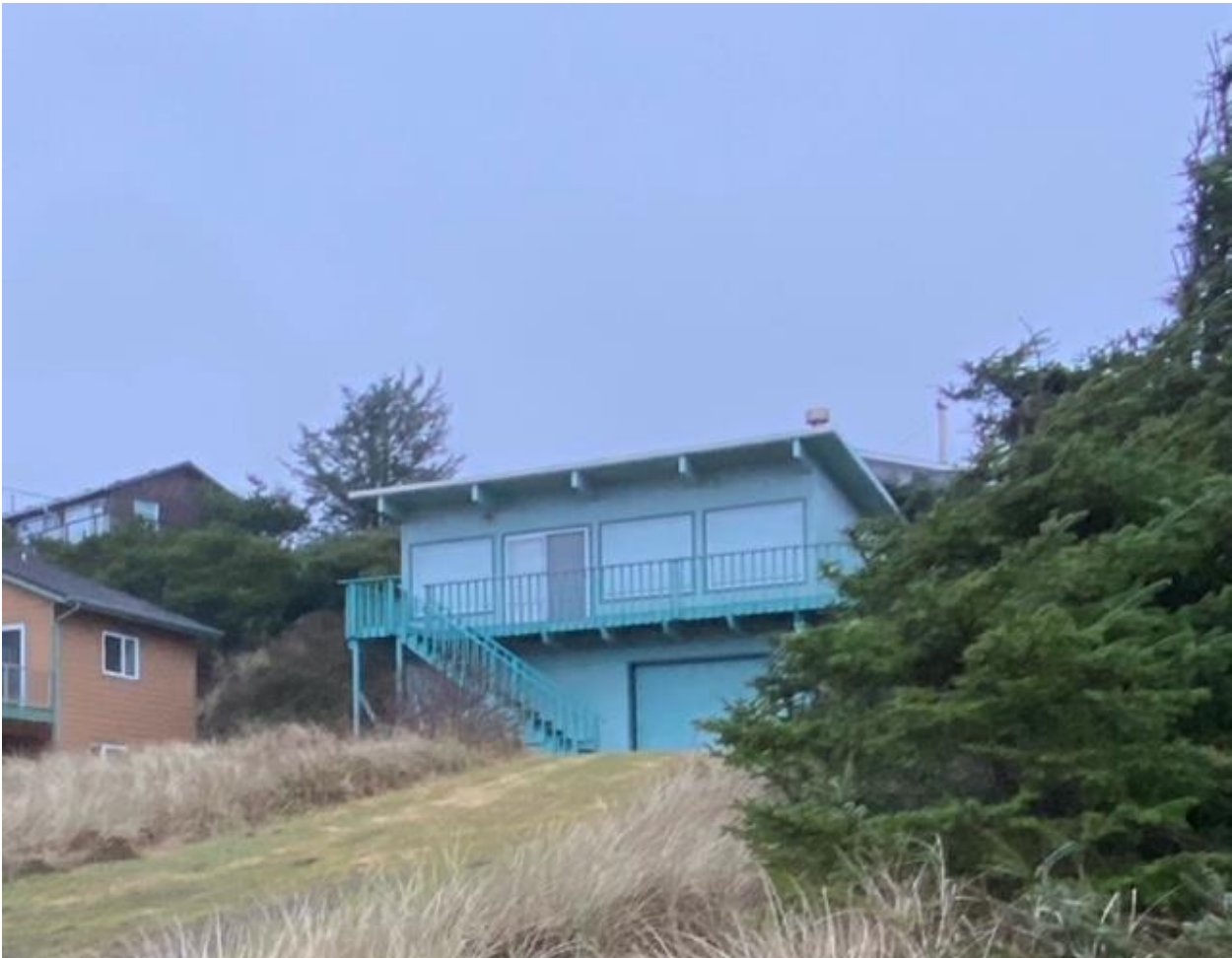
Figure Recent photo of 1713 Parker with subject tree over left roof line
