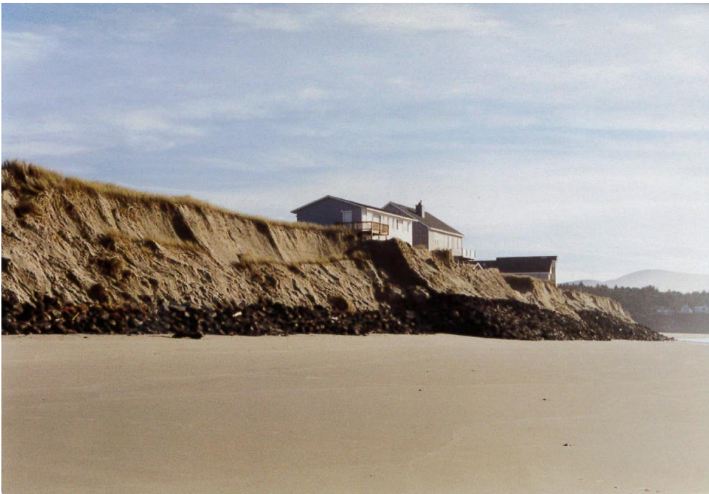
Figure 2. El Niño erosion event 1998, exposing rip-rap installed during 1984.
